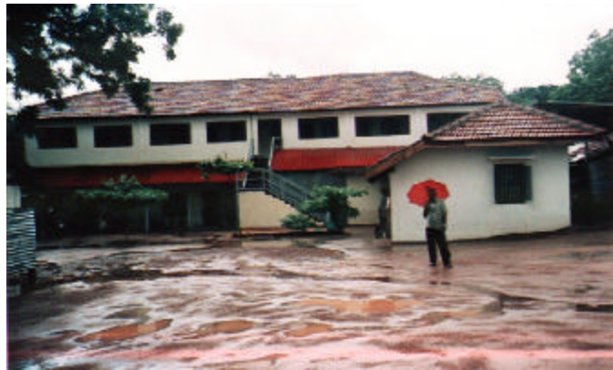
Figure 1 - Temporary Future Home of VanniTech
